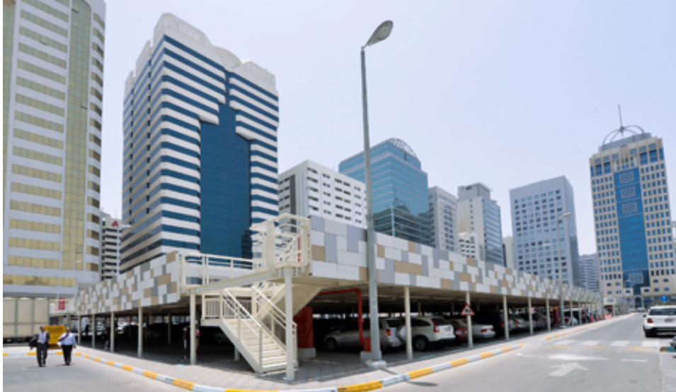
The Department of Transport in Abu Dhabi has inaugurated the first Mawaqif steel-structure car-park building in Abu Dhabi. Photo courtesy Mawaqif
